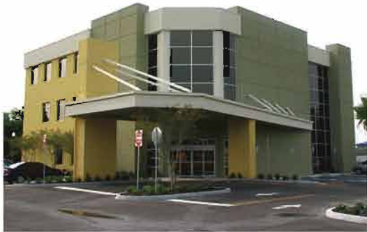
Longwood Medical Offices New Medical Construction 450 W SR 434 Status: Completed
