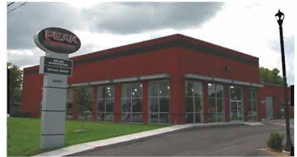
Peak Performance New Retail/Commercial Construction 2350 South US 17-92 Status: Completed
